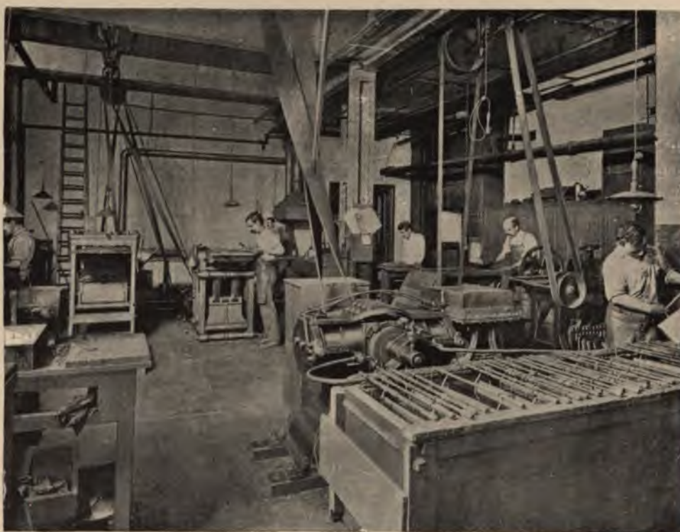
MOULDING AN ELECTROTYPE.
